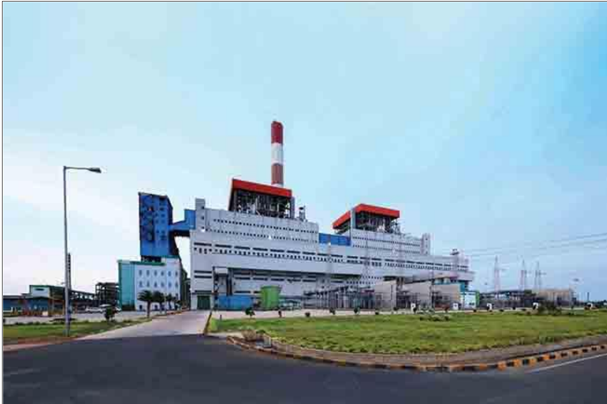
1. The SEIL Energy India Limited power plant, a 2.64-GW supercritical coal-fired facility in Andhra Pradesh, India, features four 660-MW units that deliver high operational efficiency, advanced emissions control, and innovative seawater cooling systems. Courtesy: SEIL
